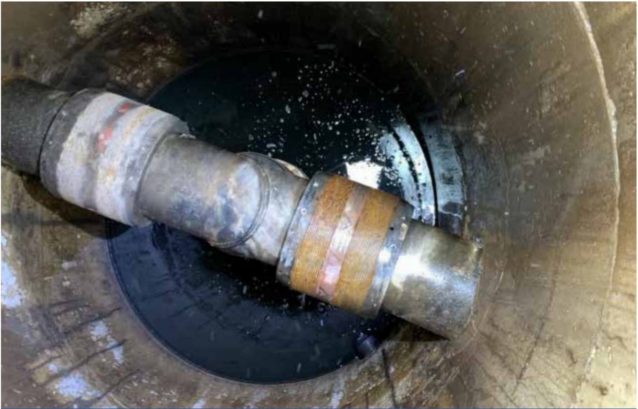
REPAIRS TO A LEAK IN THE BIOGAS EXTRACTION SYSTEM
