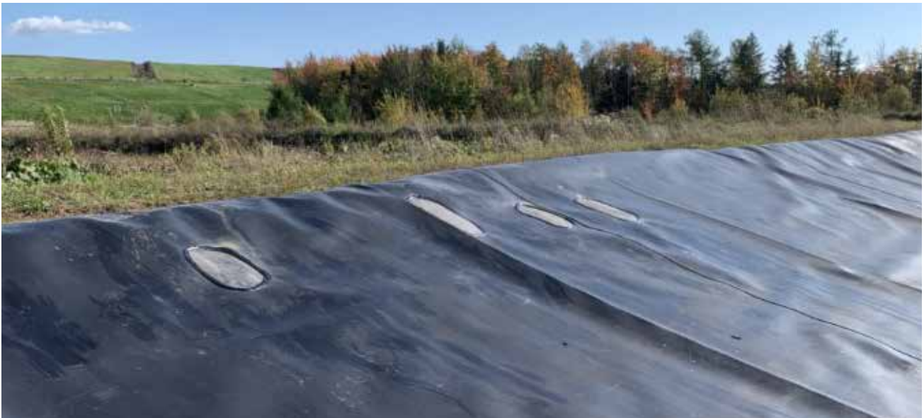
REPAIRS TO THE GEOMEMBRANE LINER
