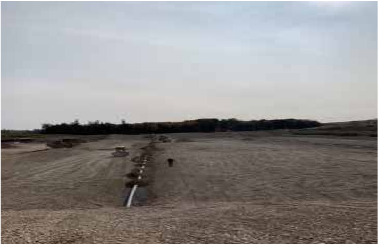
EXTENSION OF THE BIOGAS COLLECTION PIPE
